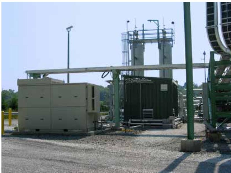
Capstone CR200 microturbine integrated with the Fallowfield Gas Processing Plant.
