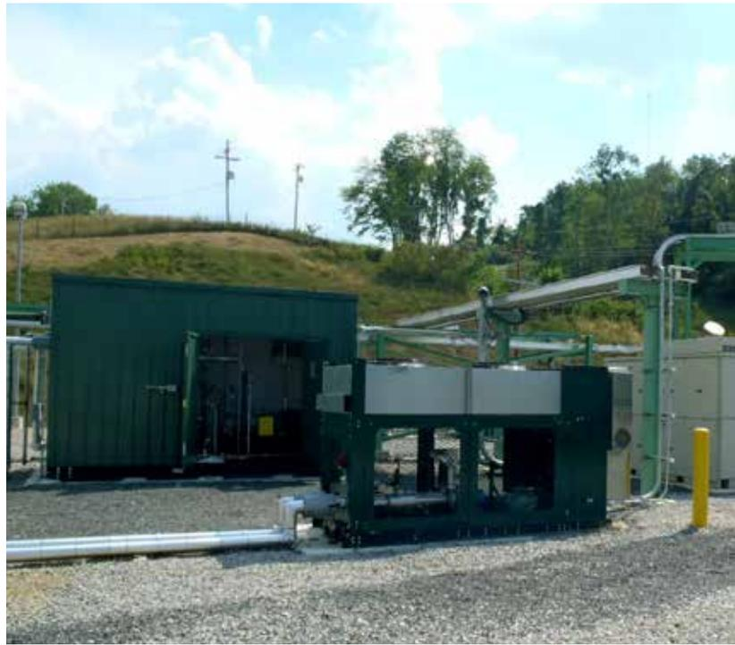
*The microturbine system includes a gas conditioning skid, chiller, and microturbine.*
