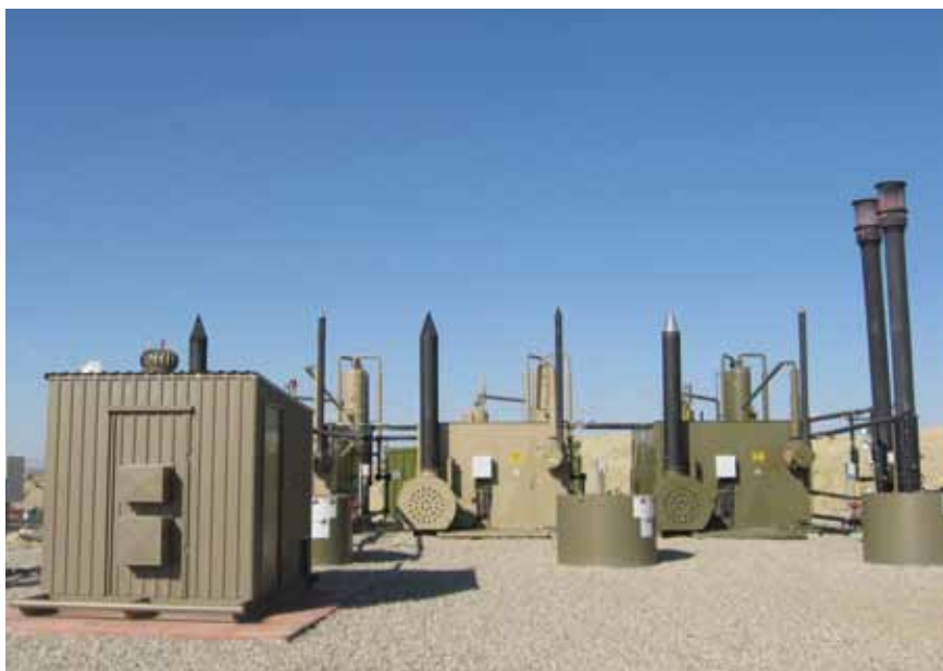
The remote Jonah Field wellsite uses a Capstone C30 microturbine to generate electricity to run the site's pumps.
