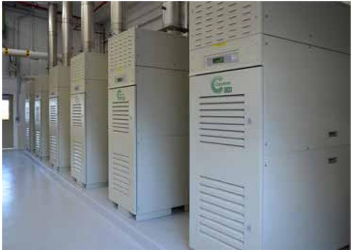
Natural gas fuels six Capstone C65 Integrated CHP microturbines that produce 390kW of clean and reliable power, as well as thermal energy for the Viking Yacht Company
