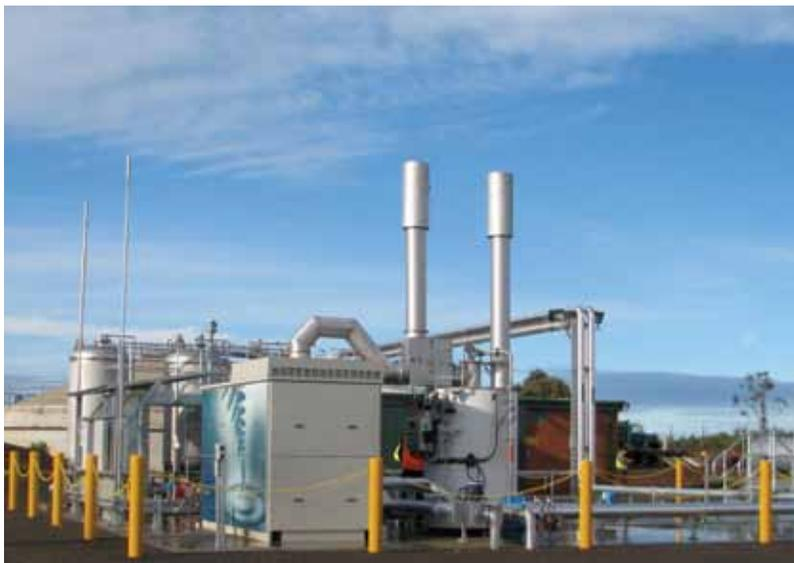
At Western Water's wastewater treatment plant in Melton, Victoria, a CR200 Microturbine burns biogas from the anaerobic digester to produce 1,700MWh of electricity each year. The electricity offsets the plant's overall power consumption by an estimated 60 percent.
