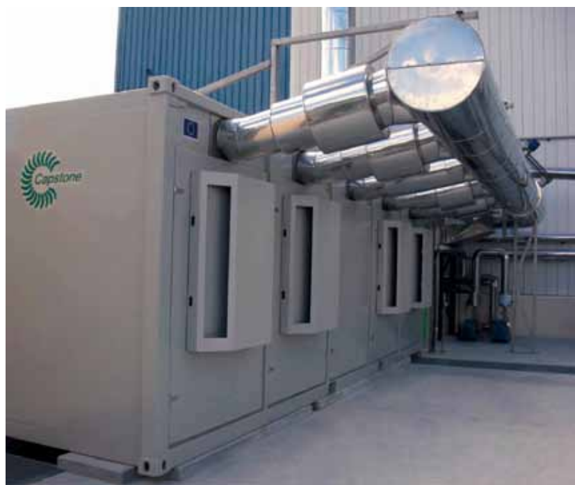
A C800 Power Package is fueled by methane from the treatment of sludge waste (from grape skins and stems) following the distillation of wine to make Cognac.
