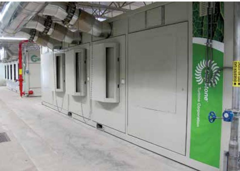
A natural gas and methane gas fueled Capstone C1000 and CR600 at York's wastewater treatment plant save energy, cut operational costs and protect the environment by generating clean-and-green electricity.
