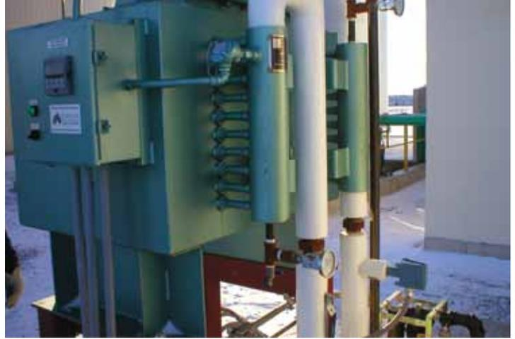
*Cain Heat Exchanger for heat recovery from the Capstone microturbine.*
